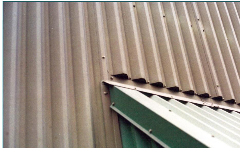
**Figure 2:** Mine smelter building exterior. Base edge and 45° angled cladding exposure. Nineteen years exposure in Northern Ontario.
