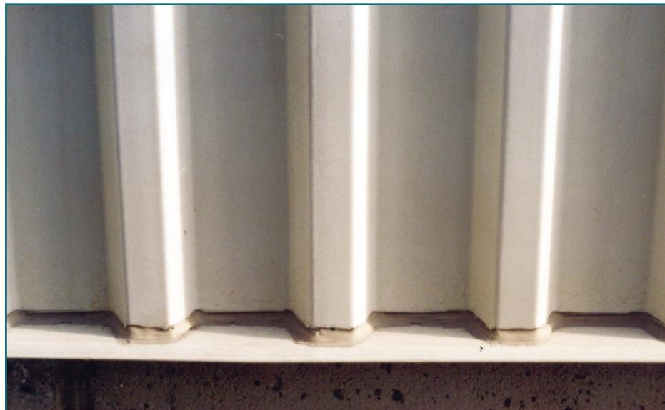
**Figure 9:** Example of effective edge sealing with caulking on an exterior wall.
