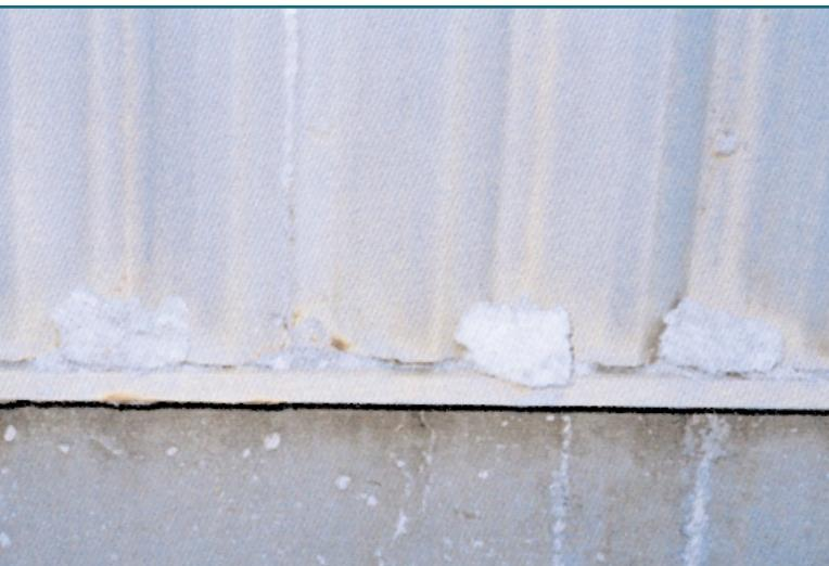
**Figure 4:** Pulp & paper plant, recovery boiler building. Ground level west exposure below exhaust duct showing contaminant build-up and minor edge creep on the cladding. Eleven years exposure in Northern Ontario.
