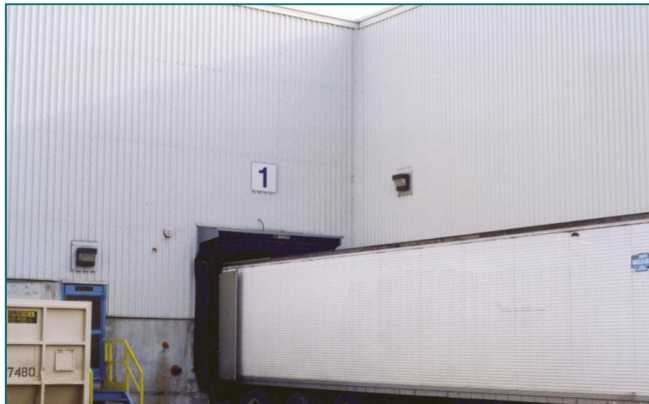
**Figure 6:** Kraft fine paper plant, paper finishing building. Comparison of new and old nine-year cladding. The newer cladding is on the right. Location in Northern Quebec.
