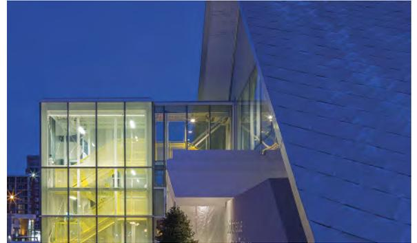
Both the spire and the roof were stripped and re-clad with Galvalume Plus™ corrosion resistant steel, arranged "à la Canadienne", in an overlapping 45-degree pattern. The attractive bright appearance and reflectivity of the roof in all weather conditions is one of the new library's most striking features.
